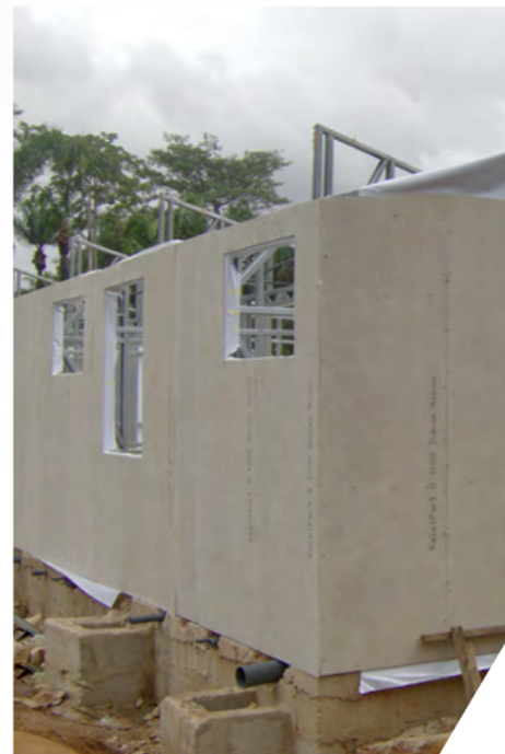
Progress on the Owerri social housing project
