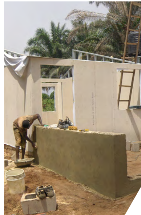
Construction of social housing in Owerri
