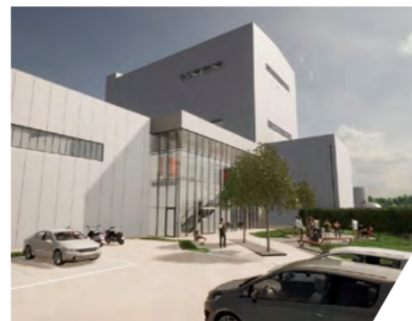
Exetex plasterboard facility expansion in Bristol, UK
