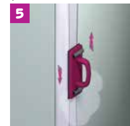
5 Apply a thin layer of jointing plaster to the top of the tape and wait until it is completely dry, sand the dry surface using a sandpaper with min. 200
